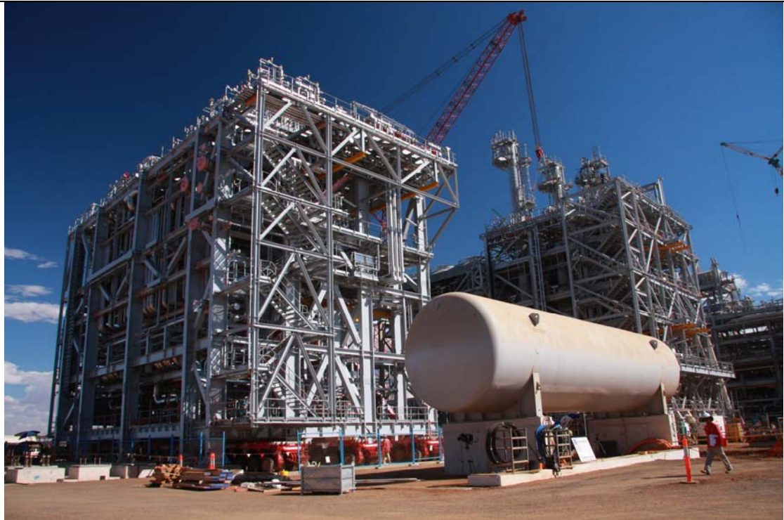
Plate 3: Final module arrives at the Pluto LNG Park, April 2010.
