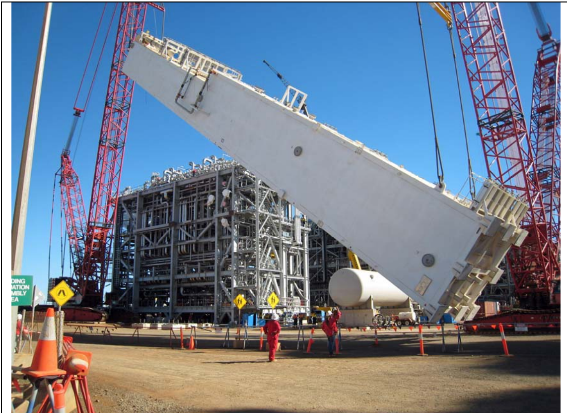
Plate 5: Final heavy lifts are completed, August 2010.
