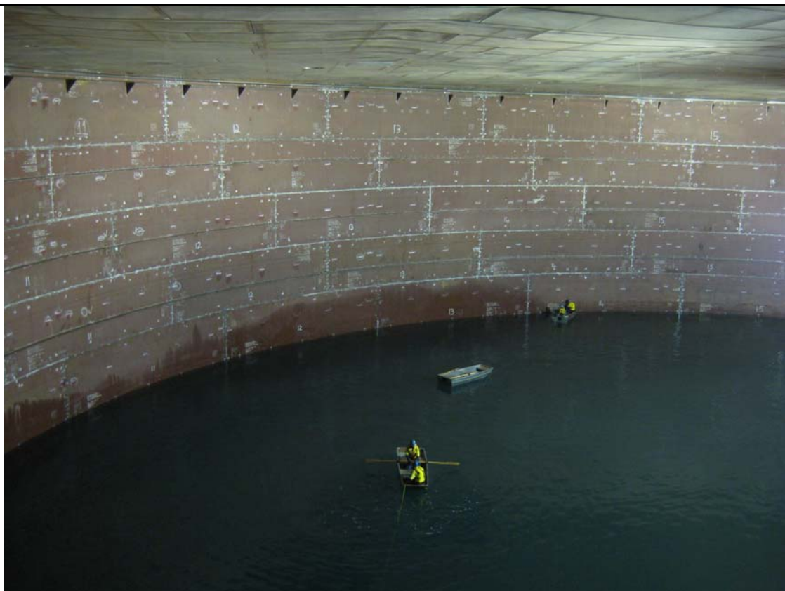
Plate 6: Hydrotesting of LNG Storage Tank 1, August 2009.
