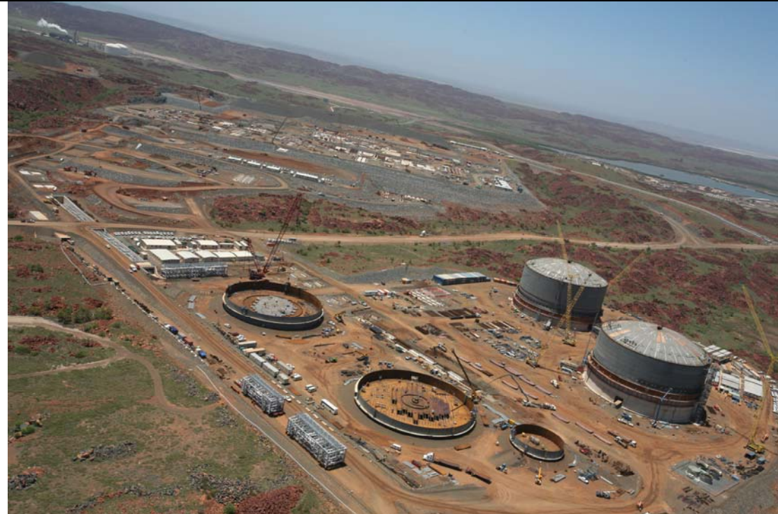
Plate 1: Pluto construction works have continued throughout 2009.
