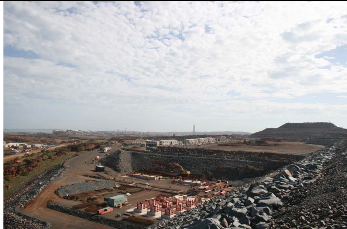
Plate 2: Site B preparation for liquefaction module arrival, February 2009.
