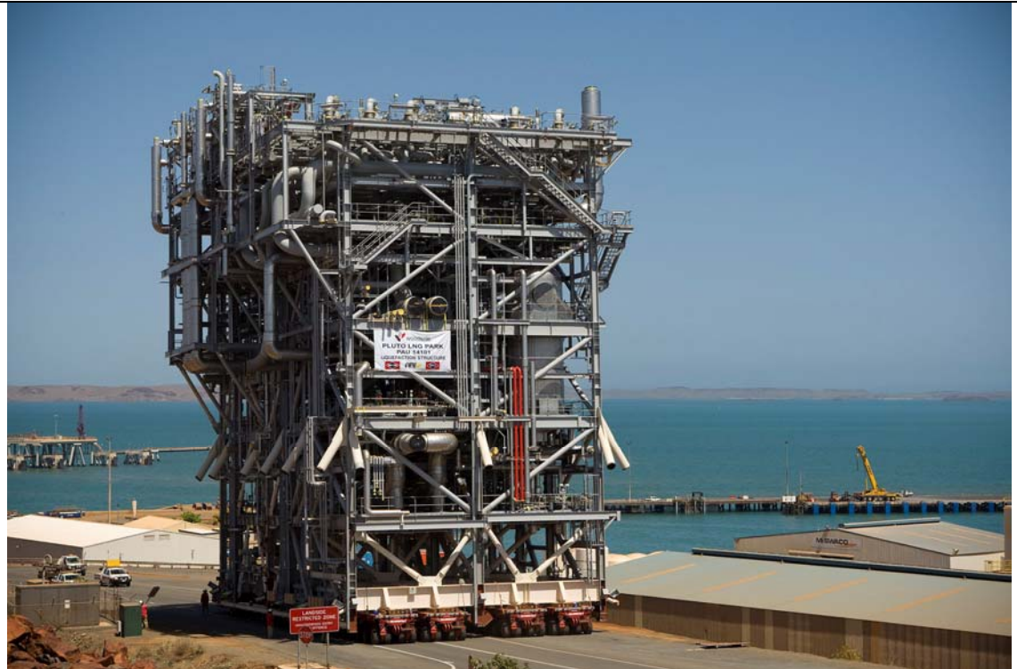
Plate 7: Arrival of largest liquefaction module (PAU 14101), 21 October 2009.
