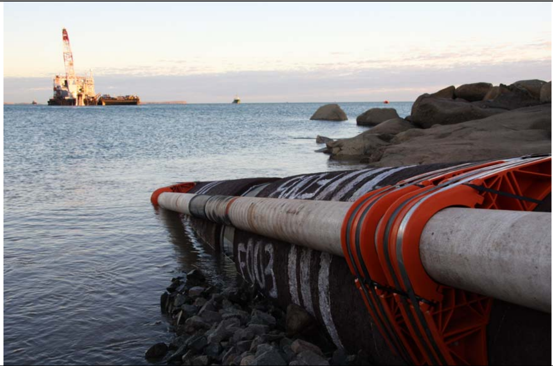
Plate 3: Pipeline shore pull, completed in May 2009.
