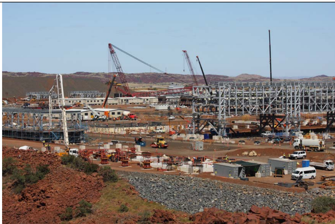
Plate 4: Module installation on Pluto Site B, May 2009.
