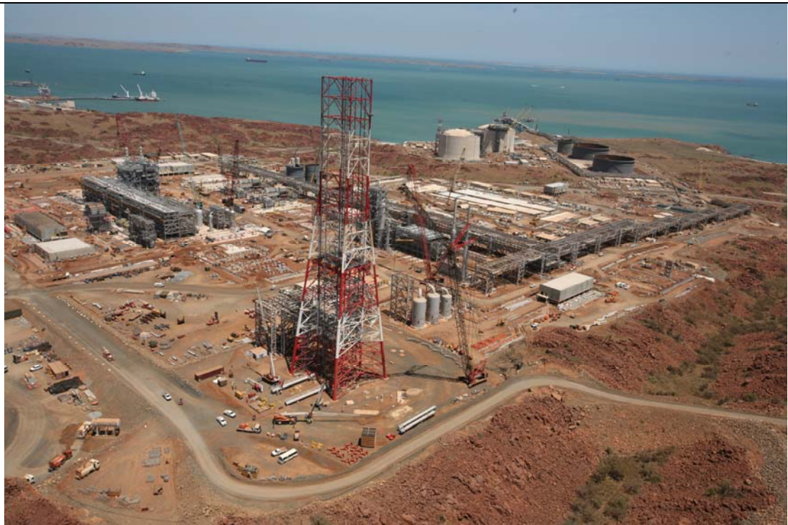
Plate 8: Flare tower construction, October 2009.
