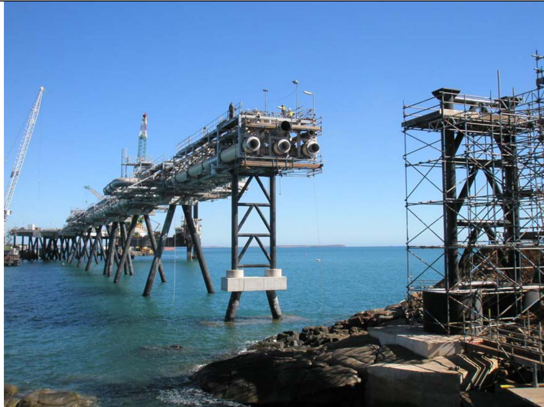
Plate 5: Jetty construction commenced in April 2008 and has continued throughout 2009.
